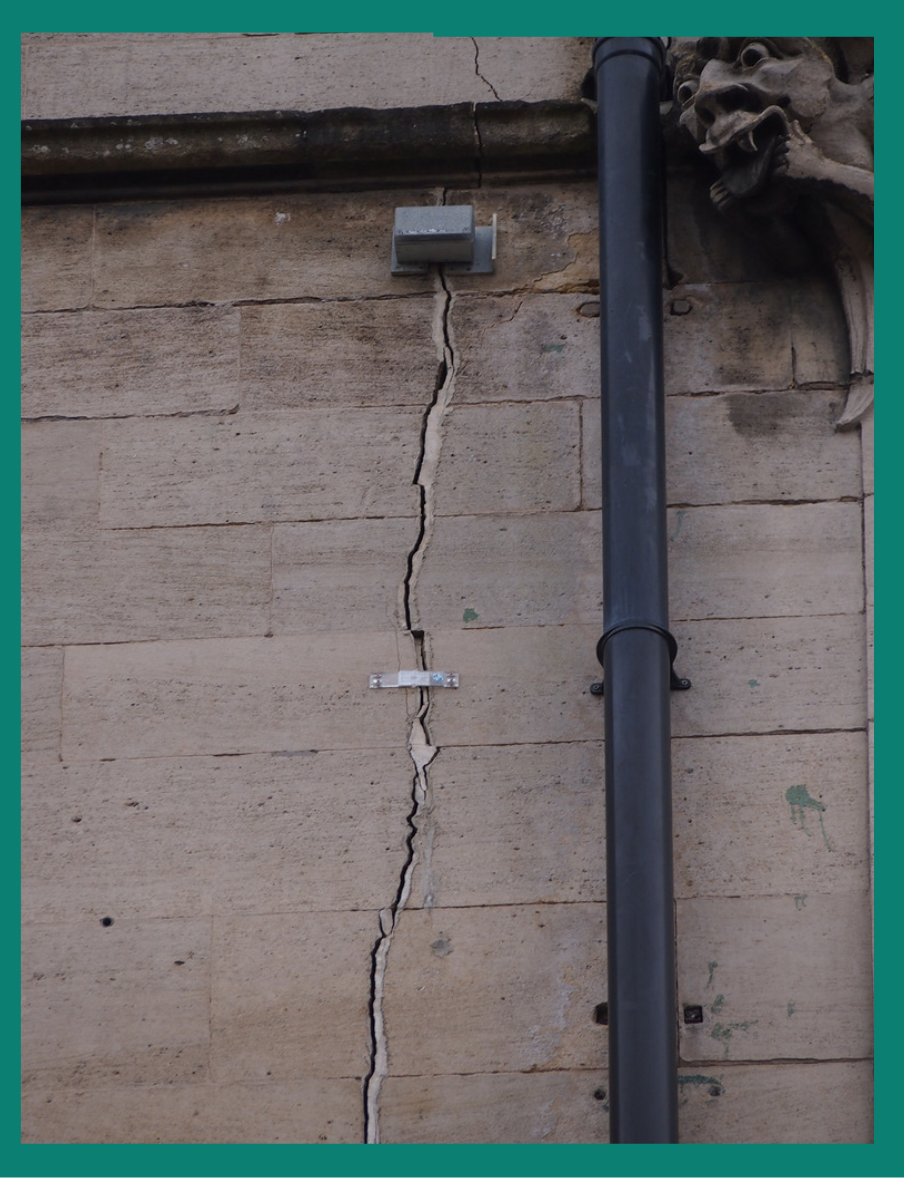
Cracks in tower and windows
