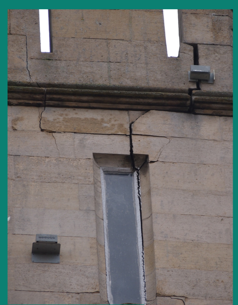
Cracks in tower and windows
